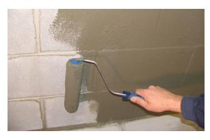
Ash Grove Pro® Wall – Tite Unsanded is a polymer modified, waterproof cement coating for above and below ground concrete and masonry surfaces. Ash Grove Pro Wall-Tite Unsanded is recommended for waterproofing, basements, cisterns, foundations, reservoirs, silos, and grain elevators.
